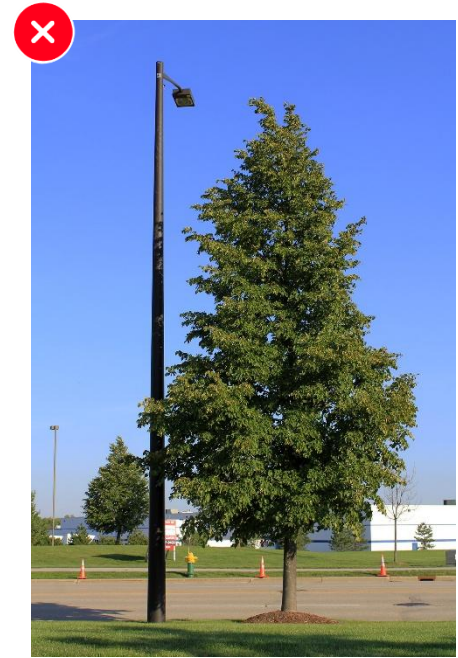
Exhibit 6-39. An example of where not to plant a tree or install a light pole
