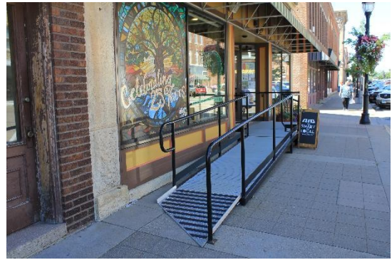
Exhibit 6-14. An example of an encroachment in a public sidewalk
