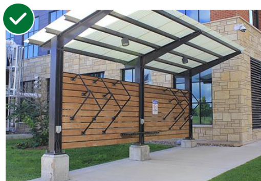
Exhibit 6-24. An example of a covered bicycle rack
